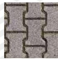
INTERNAL ROADS INTERLOCKING BLOCKS/ TREMIX CONCRETE ROAD
