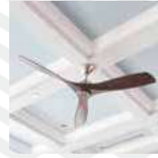
CEILING OIL BOUND DISTEMPER
