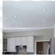
WALL / CEILING OIL BOUND DISTEMPER
