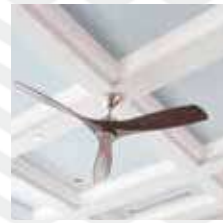
CEILING OIL BOUND DISTEMPER
